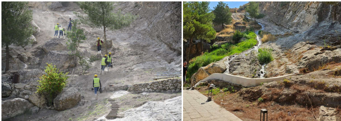
Fig. 12: artificial waterfalls that had been relocated approximately 100-200 meters away from the cave to further minimize the effects of this aspect on the entrance cave's surfaces (Before and After intervention).
