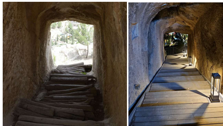
Fig. 8: Tunnel. The before and after intervention (iron and timber).
