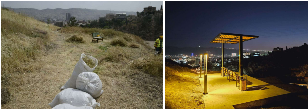
Fig. 11: Creating covered rest places which situates on the west side of the cave (Before and After intervention).
