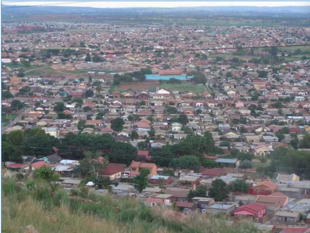
Figure 1: Aerial picture of the Mamelodi Township, CoT. Source: CoT (2023)
