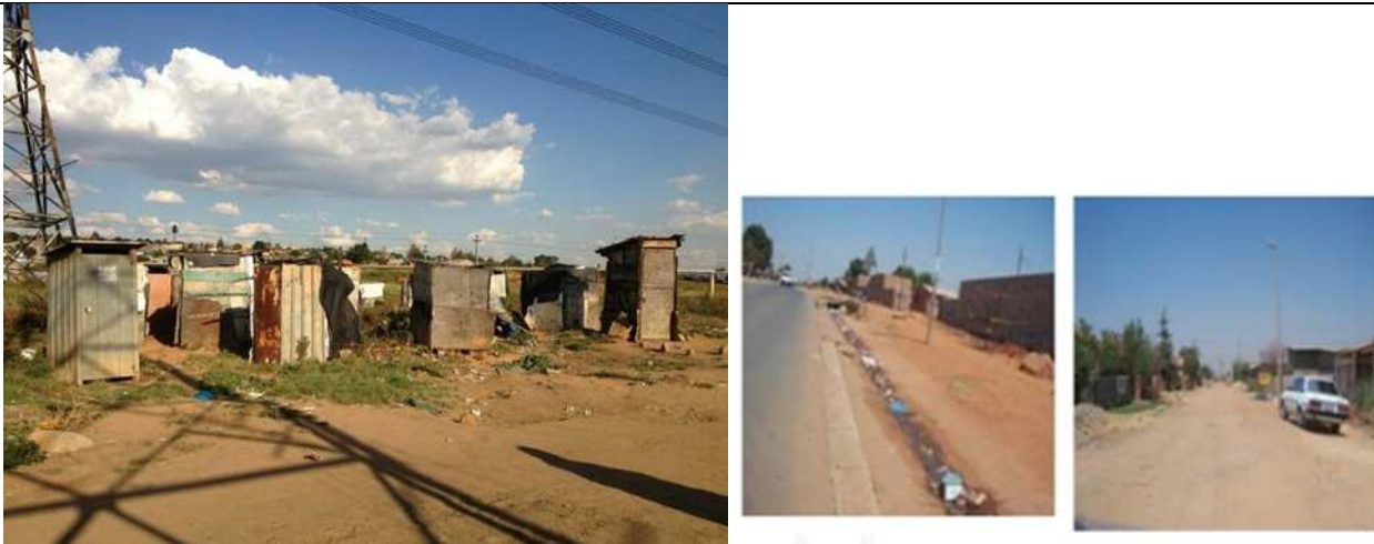
Figure 4: poor toilet infrastructure. Figure 5: States of roads in the informal settlement.
