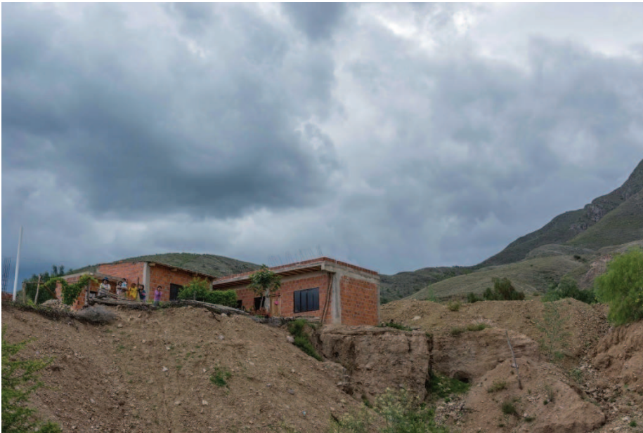
Figure 3: Housing on top of a ravine. A situation of vulnerability and environmental damage produced by uncontrolled urban expansion shaped by land speculation. Source: Author
