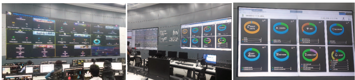
Fig 6: Inside the Integrated Command and Control Centre, Bhopal (Source: Author)
