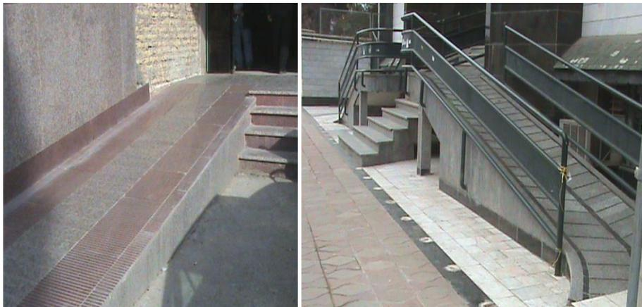
Picture 4: An entrance to a general hospital, the slope of ramp is not standard and is unprotected border. Picture 5: Ramp of inappropriate slope for access into a clinic.
