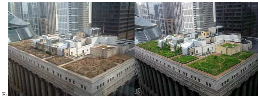
Fig.1. Green roof of Chicago City Hall, Illinois – in early spring and late summer
