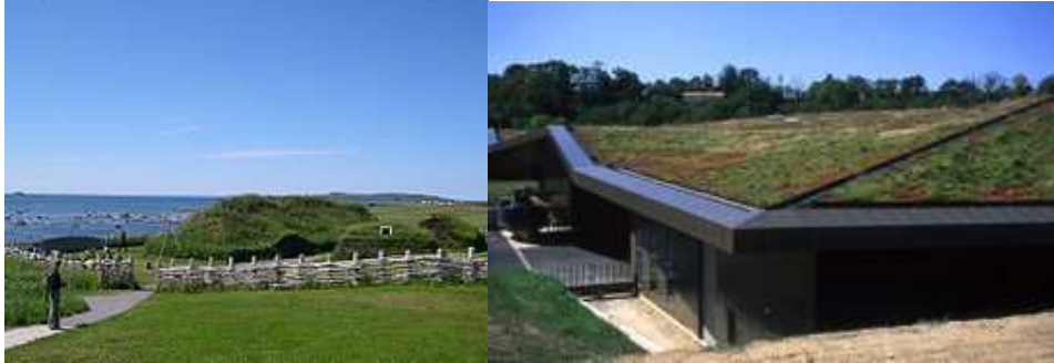
Fig.2. Newfoundland – a Wiking house Fig.3. Green roof L'Historial de la Vendée
