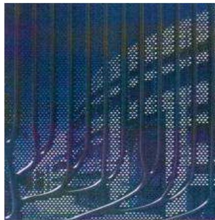
Fig.13: Transparent solar thermal facade collectors
